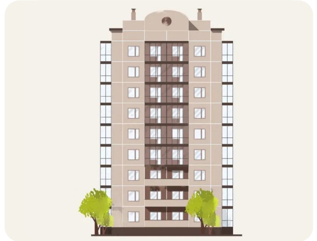
High rise building Exterior Walls
