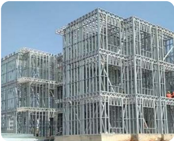
LGSF Structure Exterior Wall Houses
